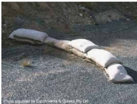
Sandbag sediment trap
