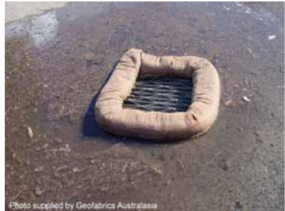
Filter sock drop inlet protection
