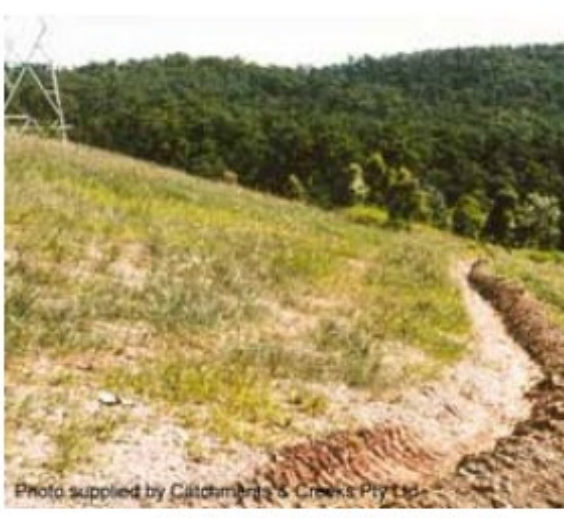
Earth-lined catch drain
