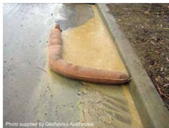
Filter sock sediment trap
