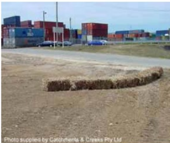
Straw bale flow diversion bank under construction (yet to be staked)
